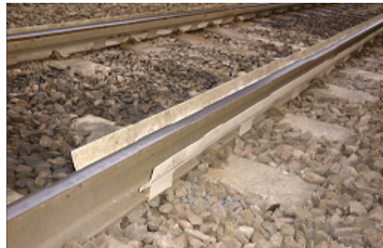
Figure 2.18 Leaf guards on the track to prevent leaves on the track.
